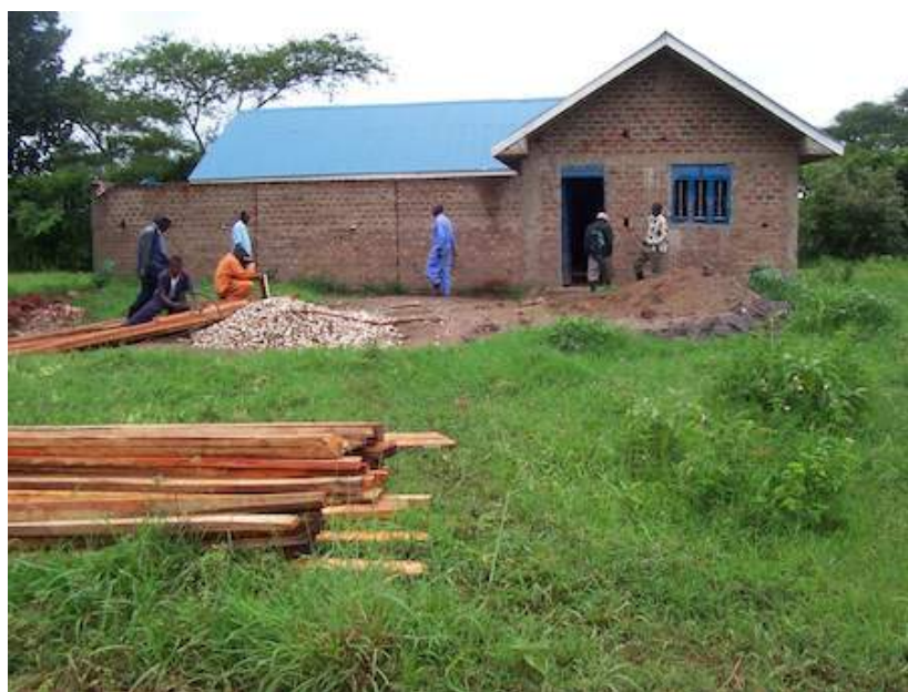
House of HOPE nearly completed in Kibogo Village
